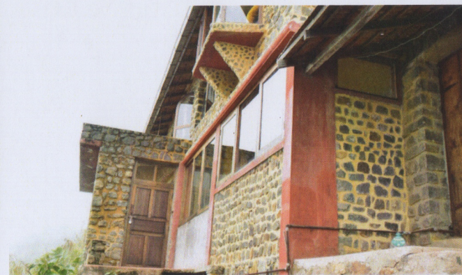
Made with stone, lime mortar and mud plaste
